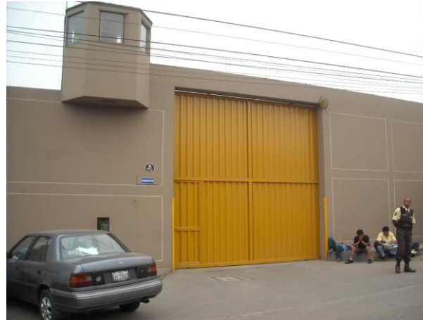
Puerta vehicular / peatonal
